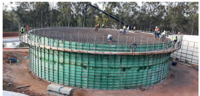
Reservoir roof steel reinforcement and formwork in place ready for a concrete pour
