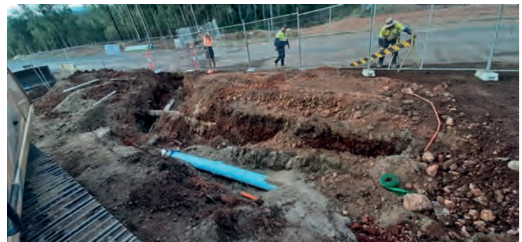
RW RM replacement after the main crosses the road (Redundant treated W main also shown)
