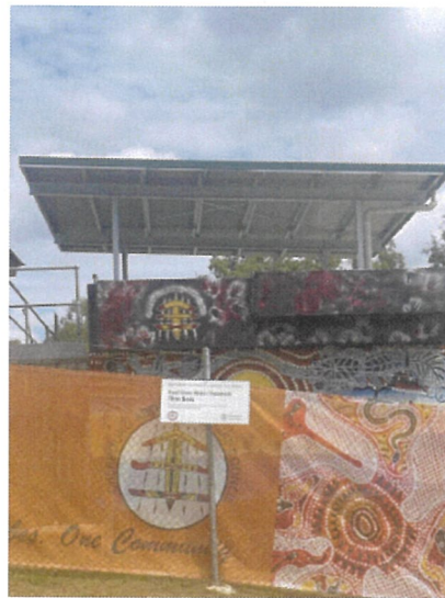
New cover over WTP Chlorinator 2024.
